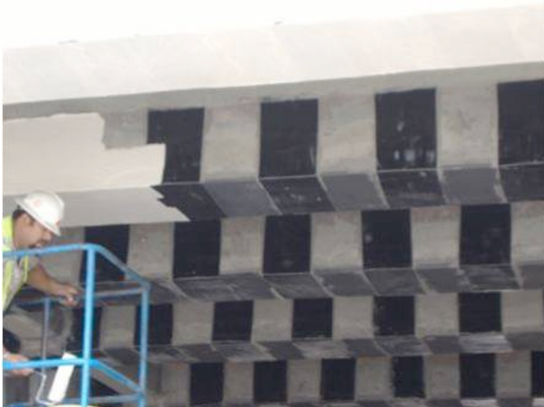
FRP used in flexural strengthening
