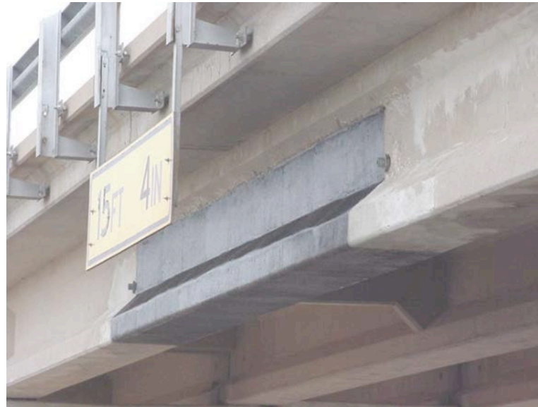
FRP used in shear strengthening
