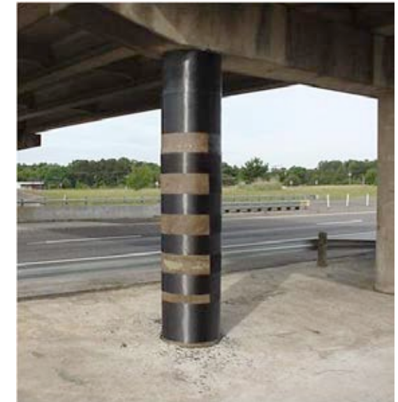
FRP used in an axial confinement
